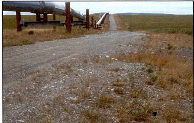
Photo 7-1. North along elevated pipeline. Gravel fill within ROW is well vegetated, except in roadway. Seeded grass and indigenous forbs predominate.
