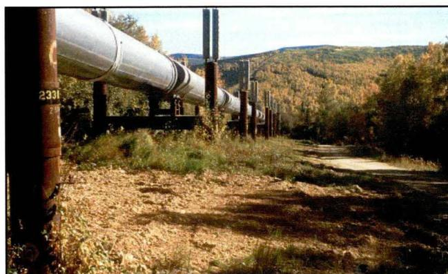
Photo 33-1. Eastward view along elevated section of pipeline. The ROW beneath the pipe has been largely invaded by trees and shrubs, which have been cut to control the growth. The roadway is largely barren. Fill has been placed between VSMs after frost bulbs raised the soil surface.
