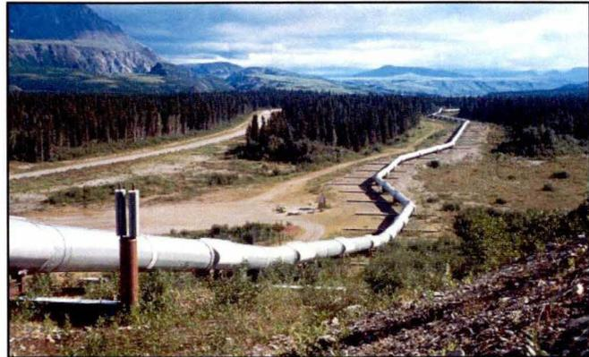
Photo 40-1. Southward view of pipeline at the Denali Fault. Gravel fill at this location is poorly vegetated, supporting only a few grasses. Wheel tracks are barren in the well-used roadway. Shrubs and trees have invaded portions of the ROW without traffic and gravel fill. Mowing is probably used to control these woody plants.
