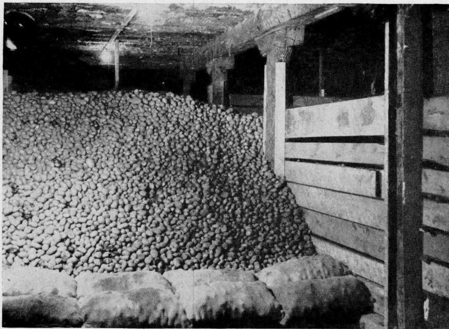
*Figure 12.*—Log construction in the earth-and-straw-covered storage.
