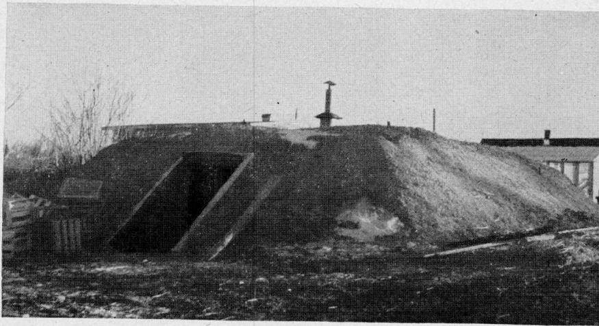
*Figure 8.*—Earth-covered storage on a level site.
