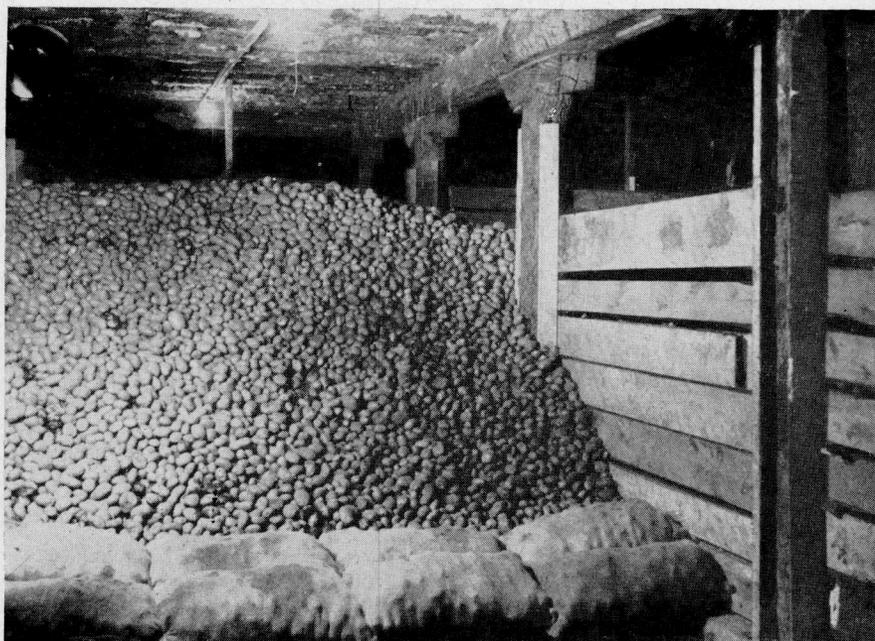
*Figure 12.*—Log construction in the earth-and-straw-covered storage.
