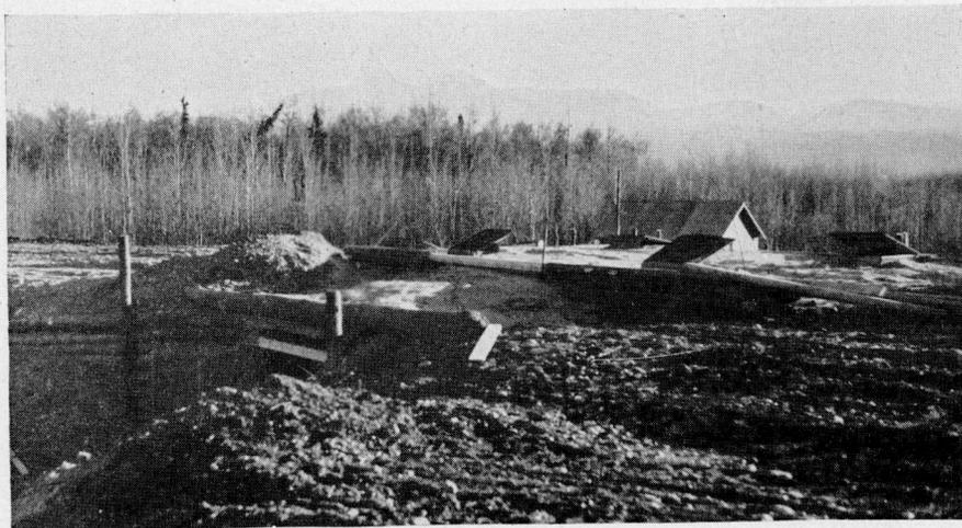
*Figure 13.*—Storage covered with 24 inches of sawdust over a log ceiling, with ceiling hatches.
