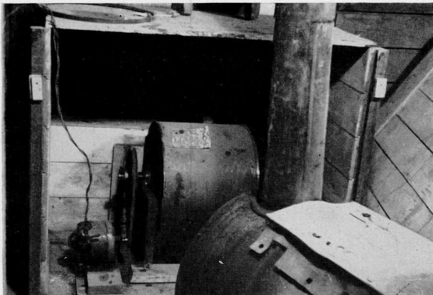
*Figure 22.*—Stove and fan chamber.
