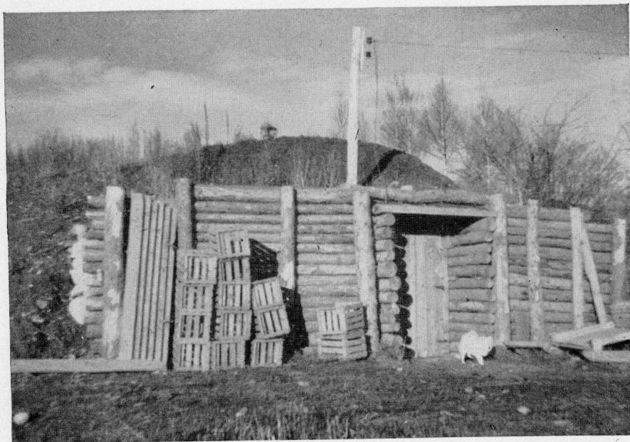
*Figure 9.*—Earth-covered storage on a bank site.
