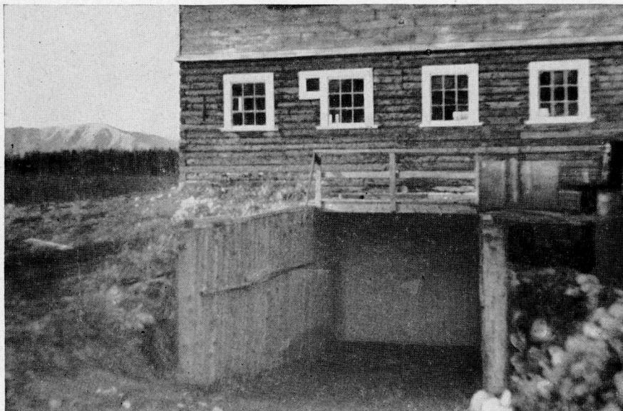
*Figure 11.*—Entry ramp to the earth-and-straw-covered storage.
