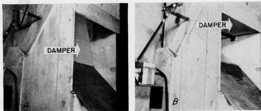
Figure 24.—Motor-and-spring-operated damper for ventilation and recirculation of air in the station storage.
