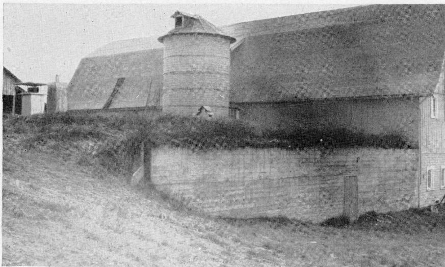
*Figure 19.*—The earth-covered concrete storage of the Matanuska Experiment Station.
