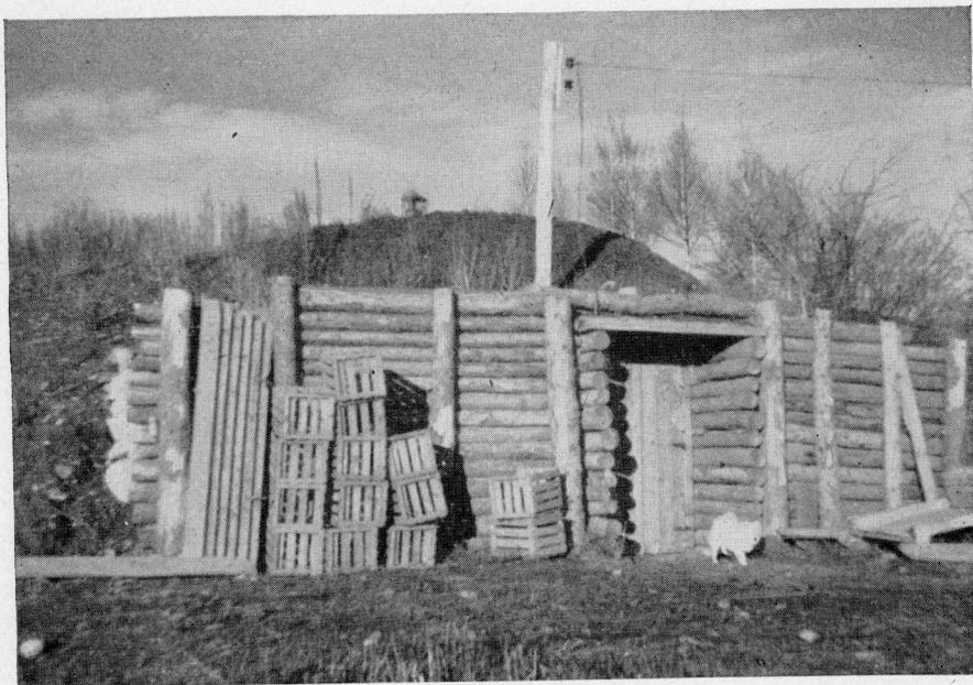
*Figure 9.*—Earth-covered storage on a bank site.
