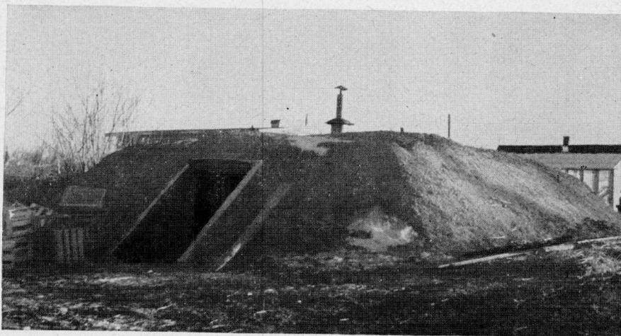
*Figure 8.*—Earth-covered storage on a level site.
