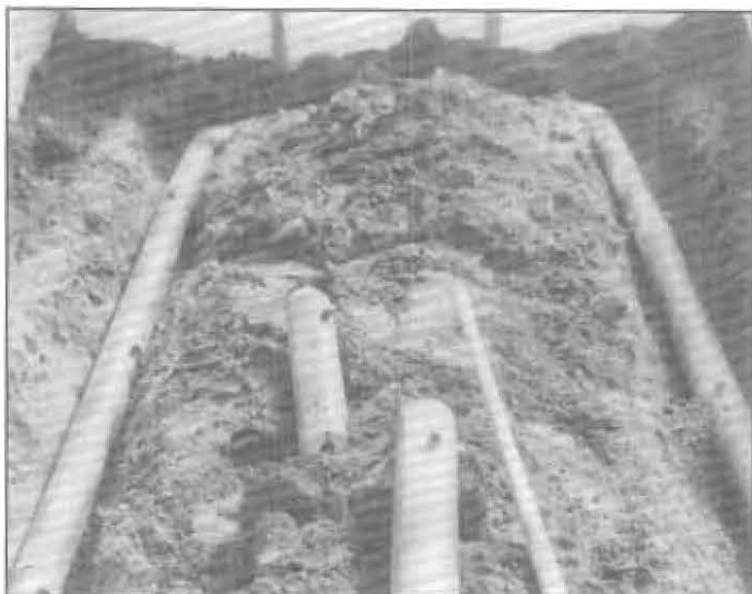
Figure 6a. Basic layout for mechanically venting exhaust air through pipes buried in greenhouse soil.
