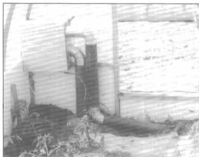
Figure 6b. A box built around a standard exhaust fan served as a manifold to accept cooled air from the soil pipes. Insulation around the perimeter retained some heat with no loss of light.
